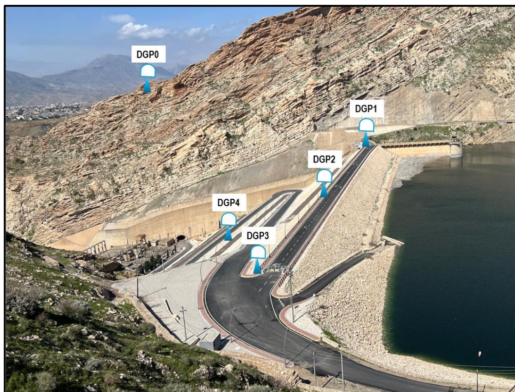
Figure 12. Deployment of the proposed GNSS receivers to monitor the movement within the dam's body.
