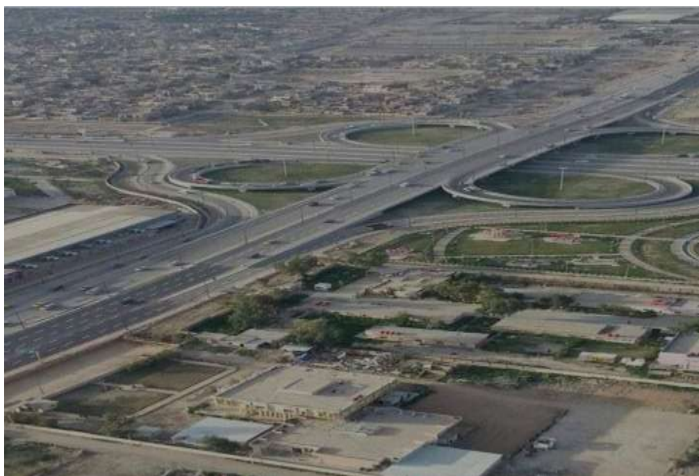
Figure 2. An aerial view from south west side of Nader Bridge in Hilla.
