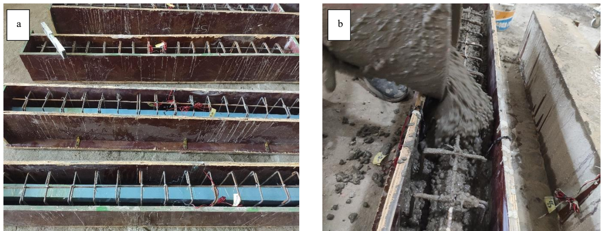
Fig. 3. Experimental work: (a); reinforcement and wooden frame (b); Concrete casting
