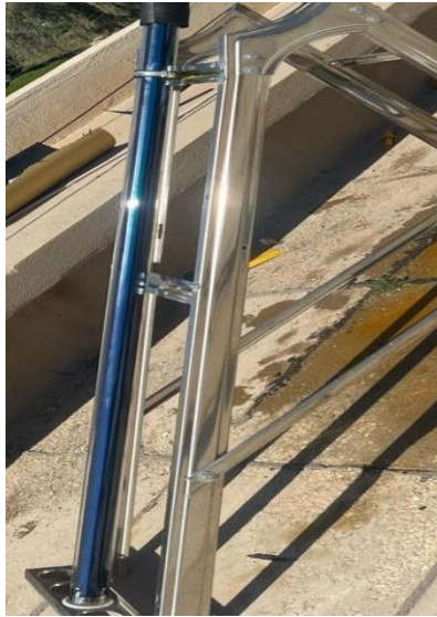
Fig. 6. The evacuated glass tube
