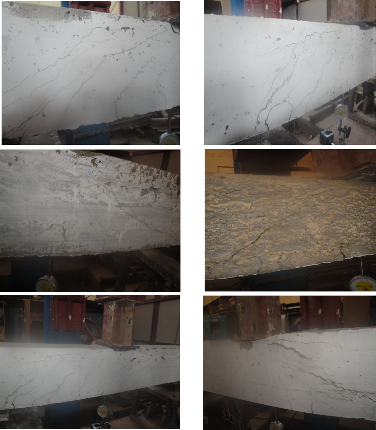
Figure 9: Crack patterns of the beams
