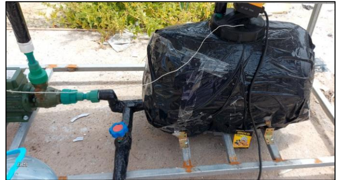
Fig. 3 The photograph of the saline water reservoir.
