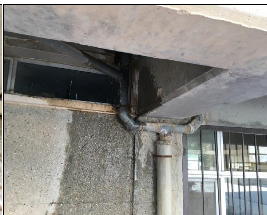
Figure 4: the old sewage pipes (2 inches
