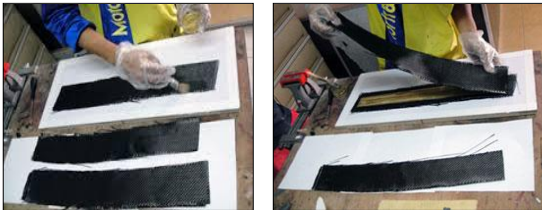
Figure 3: Typical Photographs of Composite through the Hand Layup Process.
