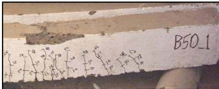
Figure (4.4) Crack pattern for strengthened beam B50-1
