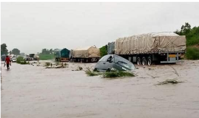
Fig. 4a: Tarred Road submerged by flood
