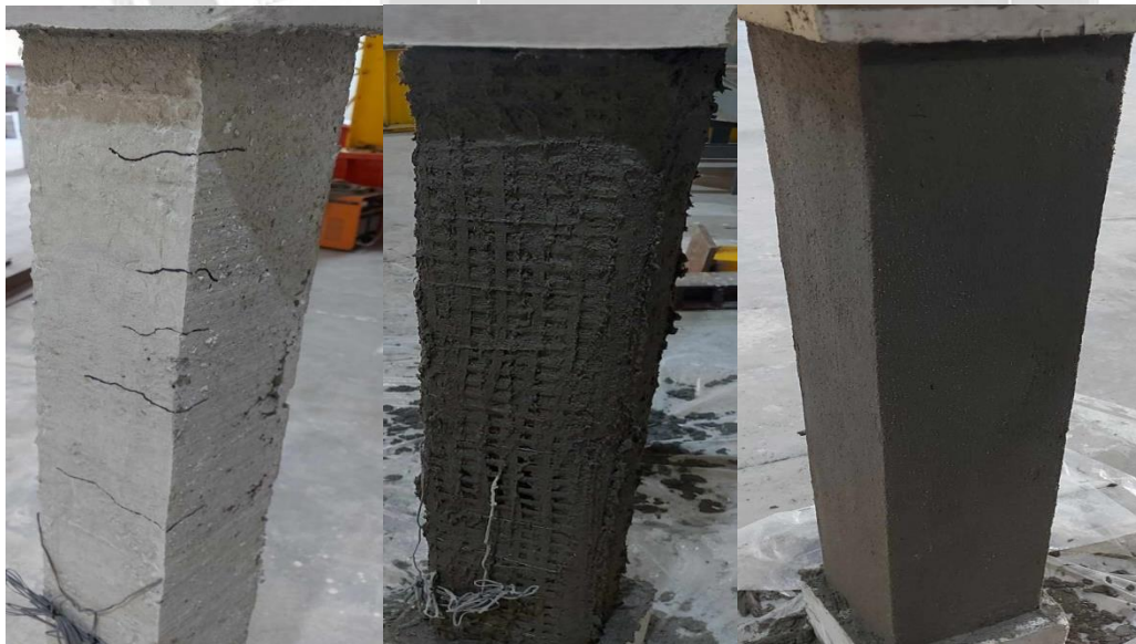
Figure (3) Retrofitting of the preloaded columns
