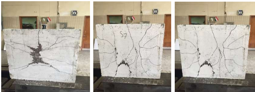
Fig 8: Cracks Pattern of Control Slab (A)
